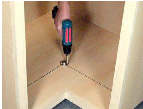
4. Mount the bottom bearing
