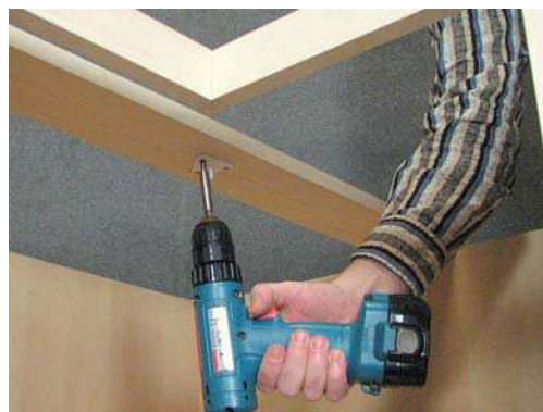
2. Screw the upper bearing
