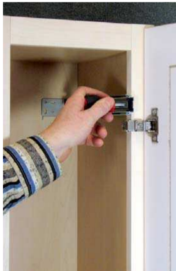
6. Screw the runner to the upper face frame
