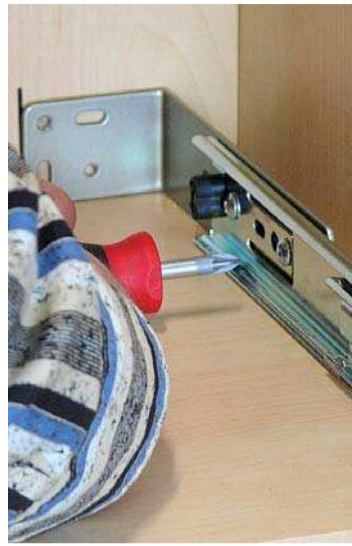
3. Adjust the required depth 4. at the runner
