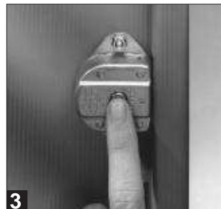
**3** Depress push-button on back of lock case and hold in depressed position.
